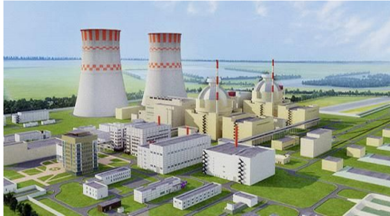
Rooppur Nuclear Power Plant
