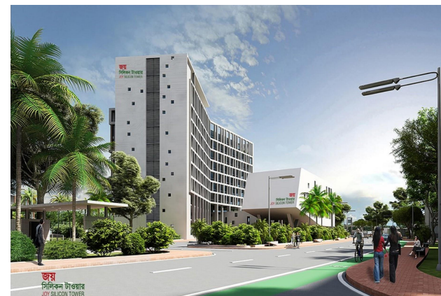
Joy Silicon Tower, Bangabandhu Sheikh Mujib Hi-Tech Park, Rajshahi
